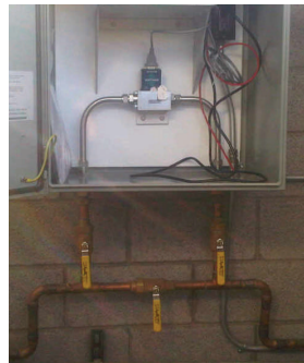
Hyperbaric split flow from a facility’s main bulk tank
